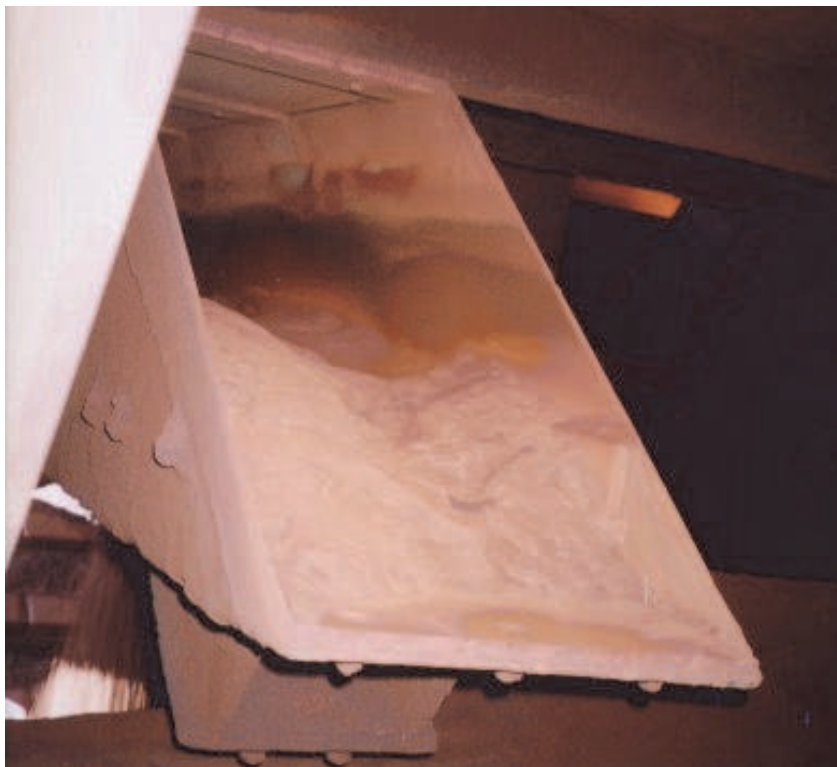
Figure 10. Partially blocked primary cutter chute.
