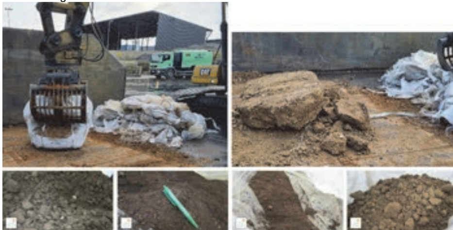
Figure 13. Ag-Au Concentrate – Discharge with crane
