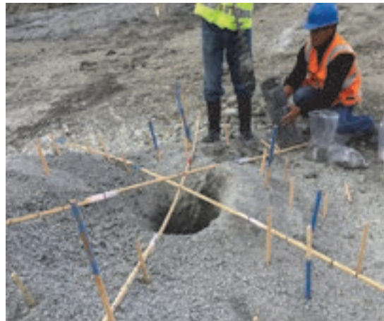
Figure 3. Reference Template sampling points over the blast hole cone
