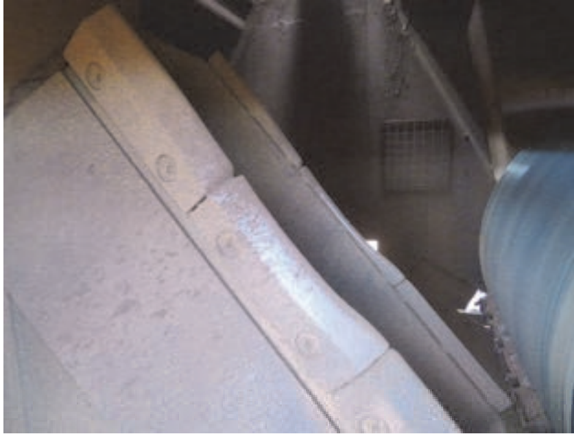
Figure 9. Primary cutter showing signs of significant wear of the cutter lips.
